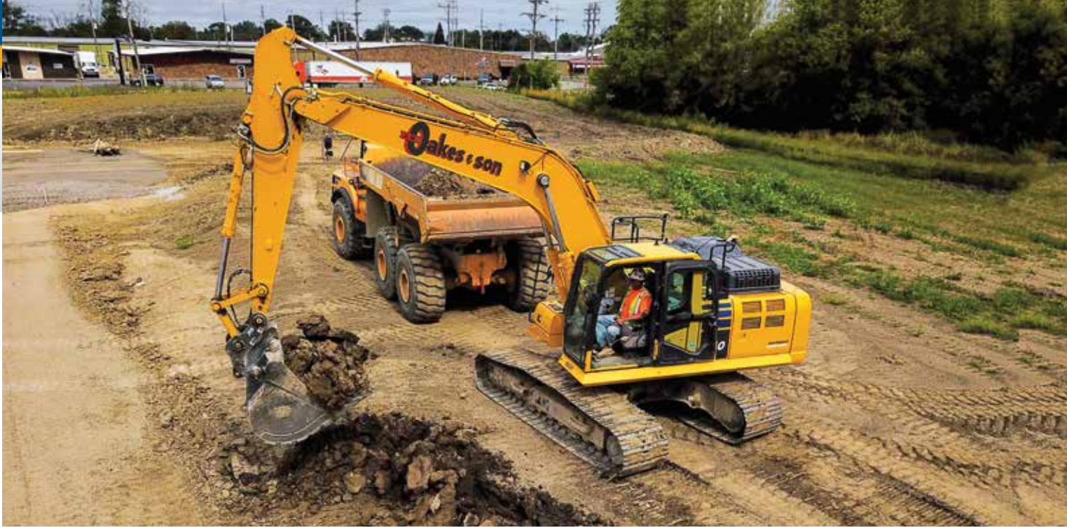
Using a Komatsu intelligent Machine Control PC210LCi excavator, an A.W. Oakes & Son operator excavates material on a jobsite in Racine. "The Komatsu intelligent Machine Control excavators are so efficient because, even as they are filling trucks, they are cutting the site to grade," stated Project Manager, Survey/Staking, Matt Krok.
