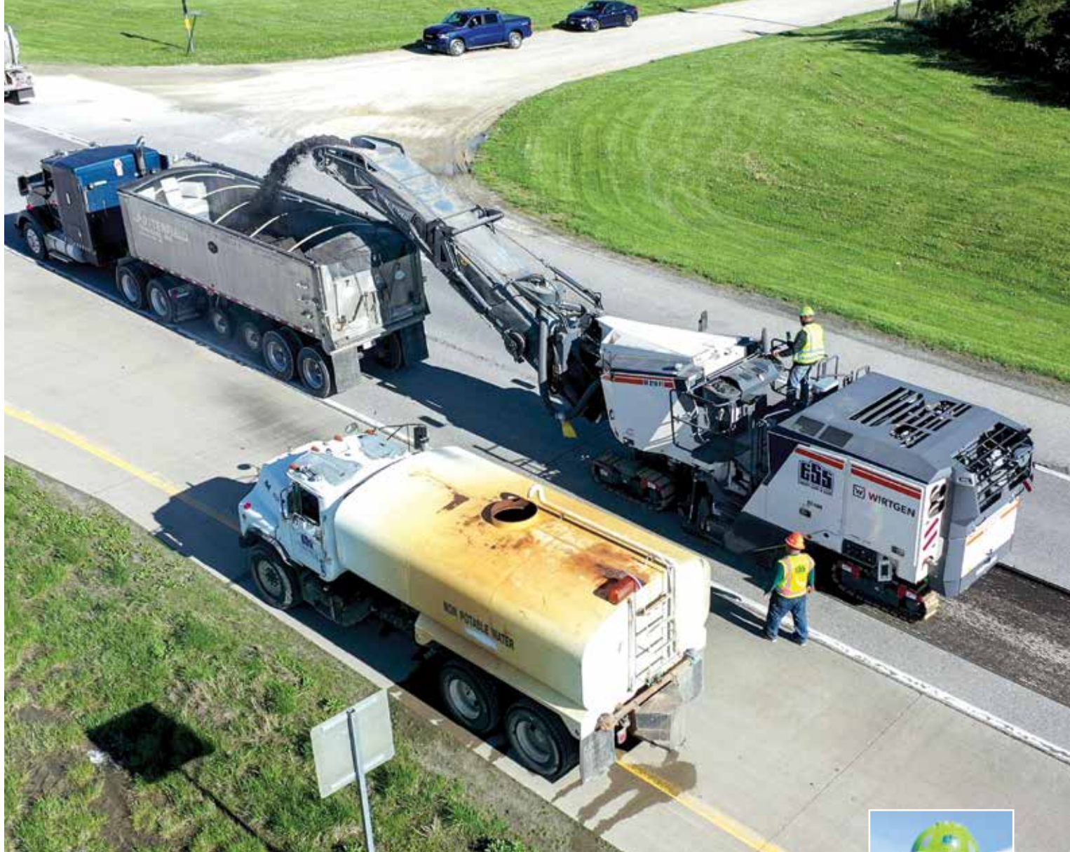
Emery Sapp & Sons' Operator Damon Dunlap uses a WIRTGEN W 210 Fi milling machine to mill an 8-mile stretch of Highway 36 near Macon, Mo. "It has more power, and I feel like it gets down the road faster. We mill hard material, but the W 210 still rides smooth."
