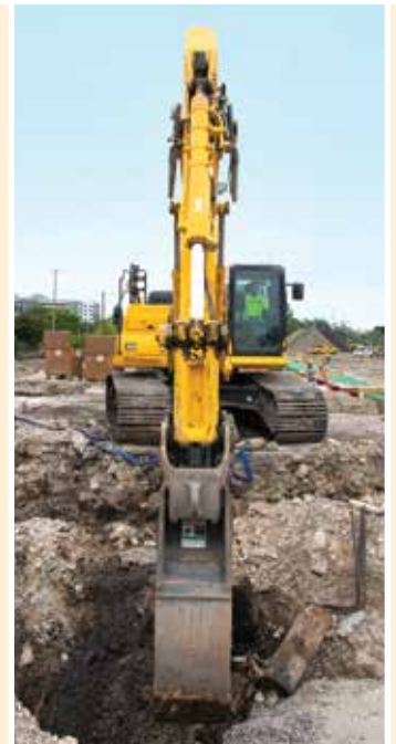
A CornerStone One, LLC operator digs with a Komatsu intelligent Machine Control (iMC) PC360LCi-11 excavator at Komatsu's future global mining headquarters. "With iMC, you can put them right to grade, and once you reach target elevation, it prevents you from overexcavating," said CornerStone One Earthwork Division Manager Scott Christman.
