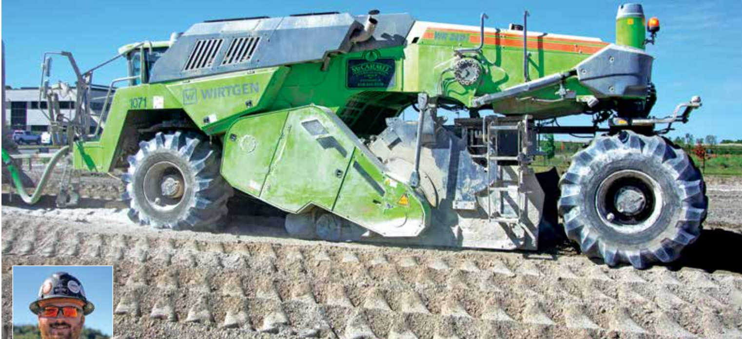
Mt. Carmel Stabilization Group relies heavily on WIRTGEN stabilizer/recyclers, including this WR 240i used to mix lime 12 inches deep with existing soil to create a firm parking lot base on a site near St. Louis, Mo. "The WIRTGEN machines are exceptional," stated Superintendent Alex Schalasky. "They outperform the competition, hands down."
