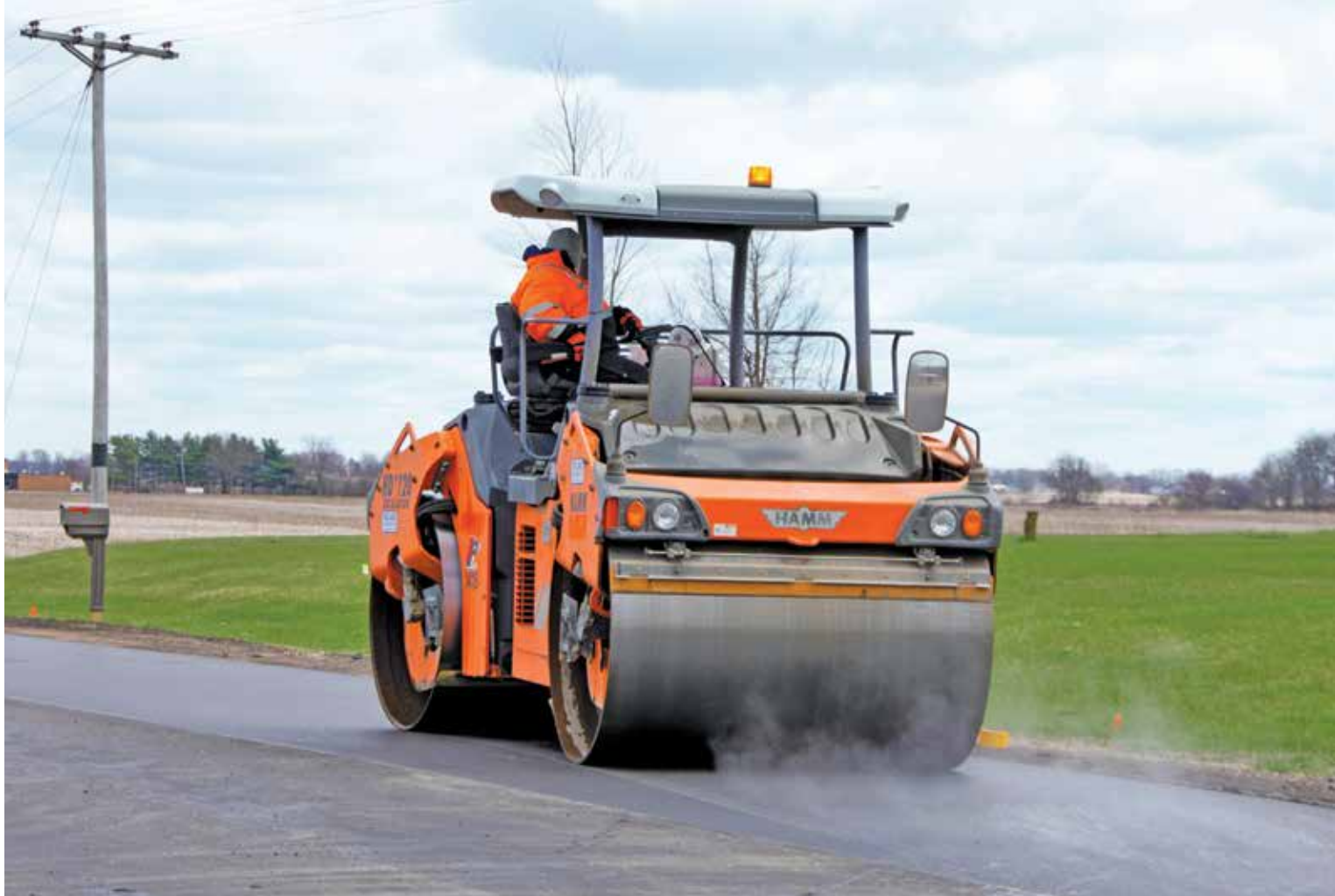
An IPC operator compacts asphalt with a HAMM HD+ 120i tandem roller.
