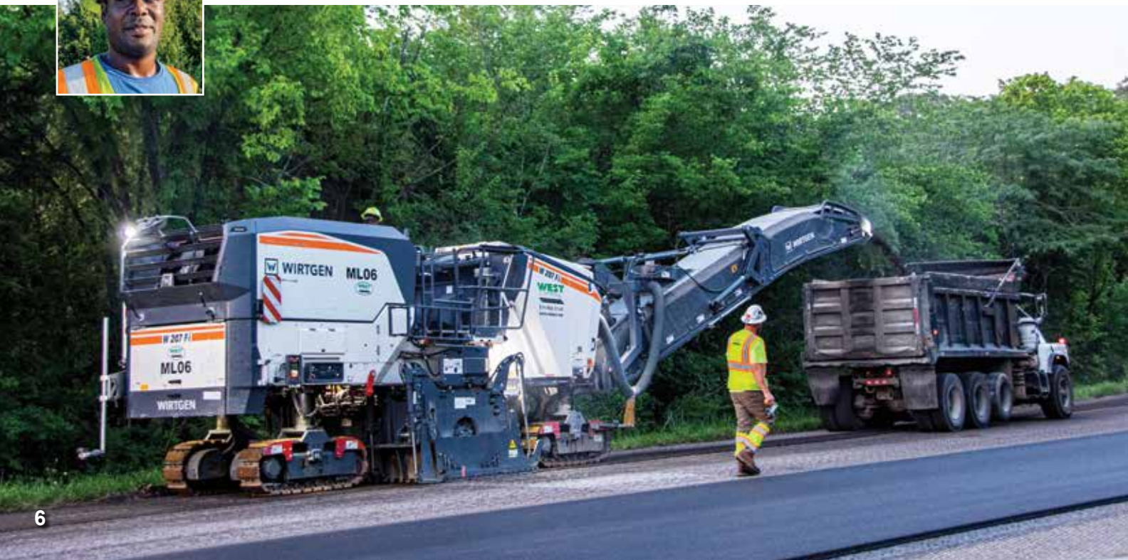
Operator Preston Shepherd uses a WIRTGEN W 207 Fi cold milling machine to load a truck with millings. "It's very user-friendly," said Preston. "If you are standing on this side, it shows you the other side of the machine, so the groundman can virtually see the other side of the machine. It has great production and power, and I would recommend WIRTGEN over any other mill."
